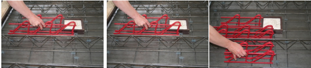
Figure 3: Installation of the FDB
