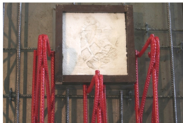
Figure 2: Installation of the FDB directly on the edge of the column
